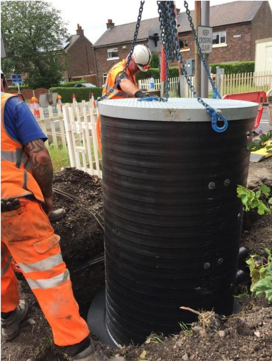
Photo: installation of an under track crossing chamber.
